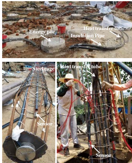
Fig. 1: Photos of construction site
